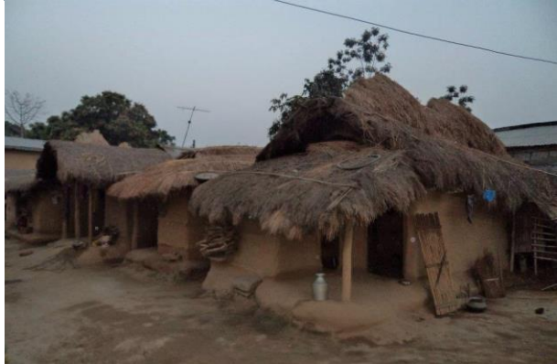
Typical mud-house of Majhi community
